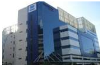
Light Industrial Buildings
